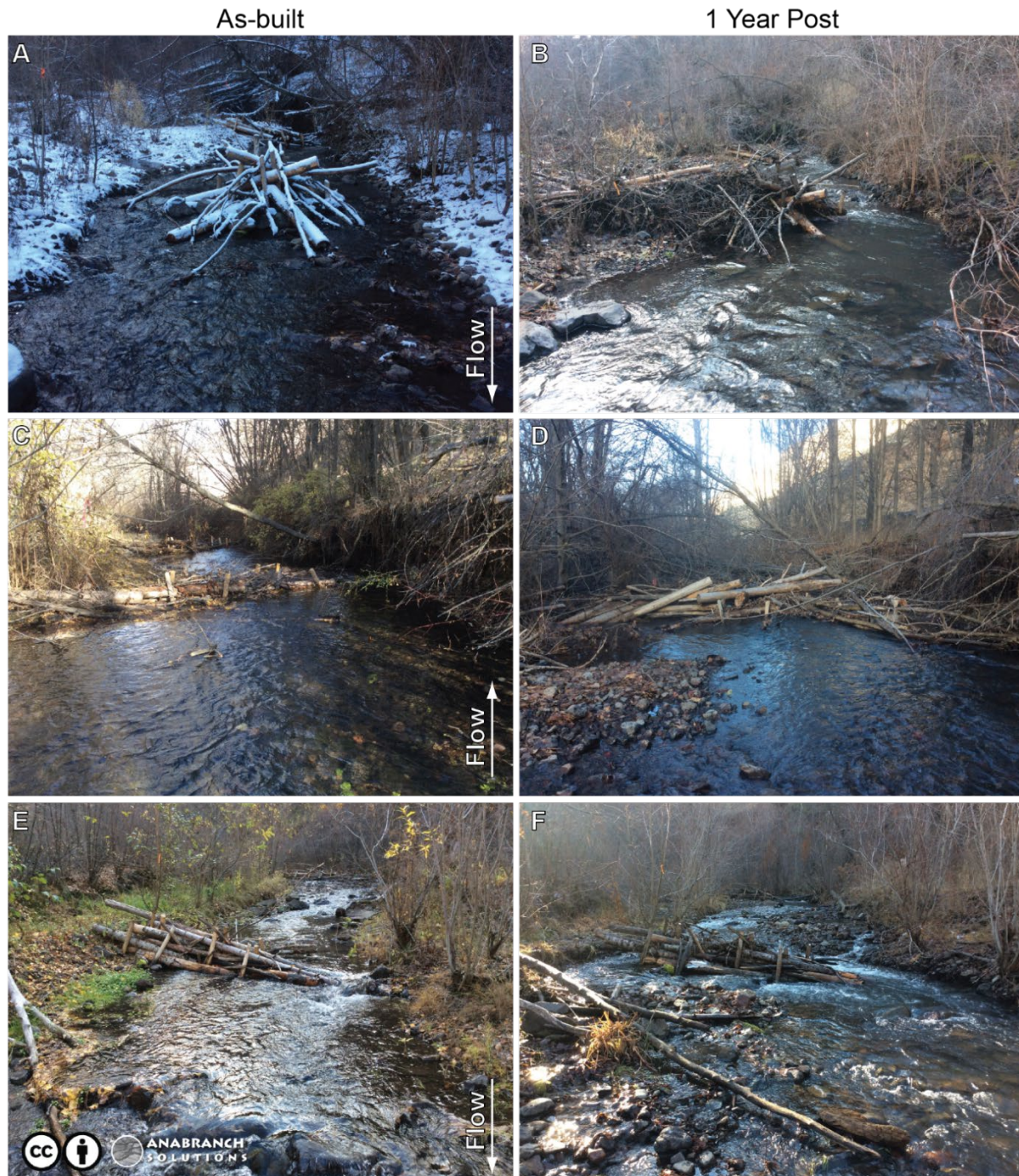
Figure 18. Example of PALS evolution over the course of one year promoting processes of wood accumulation. A and B show a mid-channel PALS becoming a bank-attached PALS, C and D show a bank-attached PALS becoming a debris jam, and E and F show a bank-attached PALS becoming a mid-channel PALS. The geomorphic changes imposed by the presence of the PALS in each example shows clear alterations to the channel bed and hydraulics. From Chapter 4 of Wheaton et al. (2019: http://lowtechpbr.restoration.usu.edu ).
