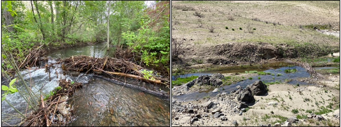
Figure 10. Example of a channel-spanning PALS after multiple years of additional wood accumulation (left photo) and a beaver dam analogue reinforced with posts (right photo).
