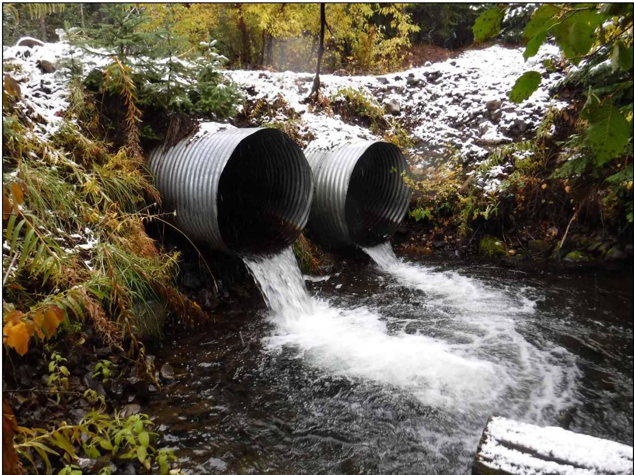
Figure 2. Existing conditions of Forest Road 80 Piscoe Creek crossing outfall.
