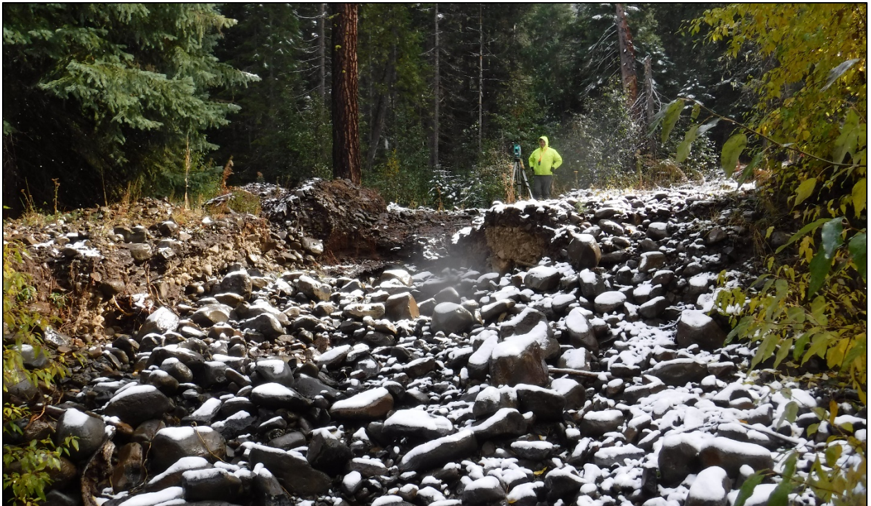
Figure 5. Road prism washout north of Piscoe Creek. Alluvial fan surface is in the foreground.
