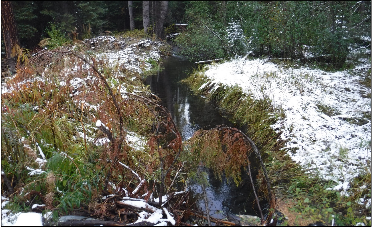
Figure 4. Piscoe Creek upstream of road crossing and culvert inlet within aggrading alluvial fan surface.
