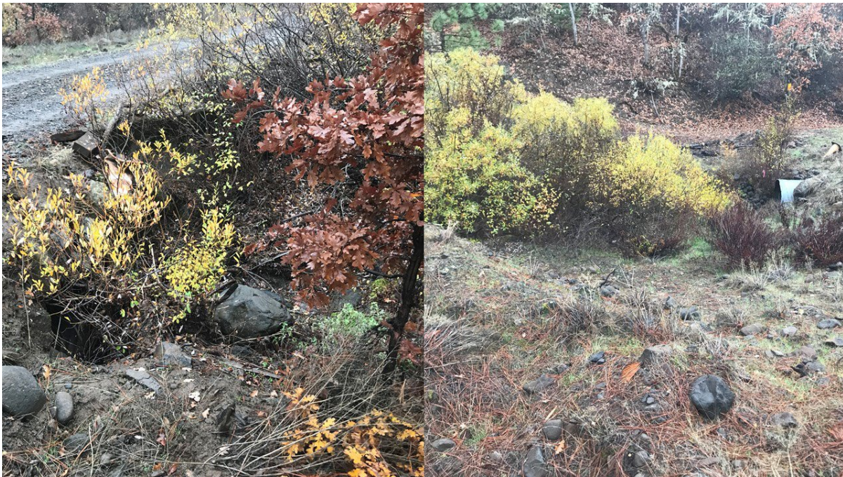
Figure 3. Photos of existing conditions of road crossings over the west (left) and east (right) tributaries.
