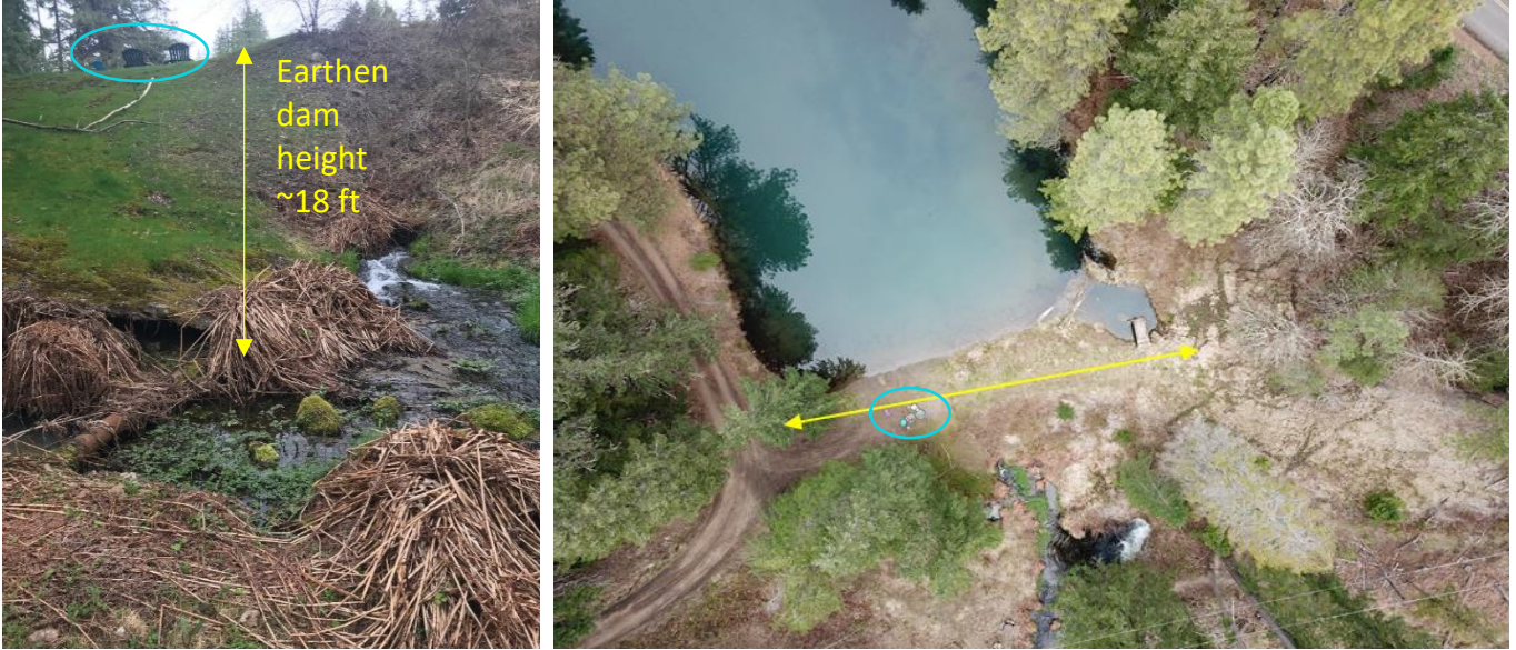
Figure 5: Dam height with small breach (L); aerial showing dam crest of 125', breach in center & overflow on right (R).
