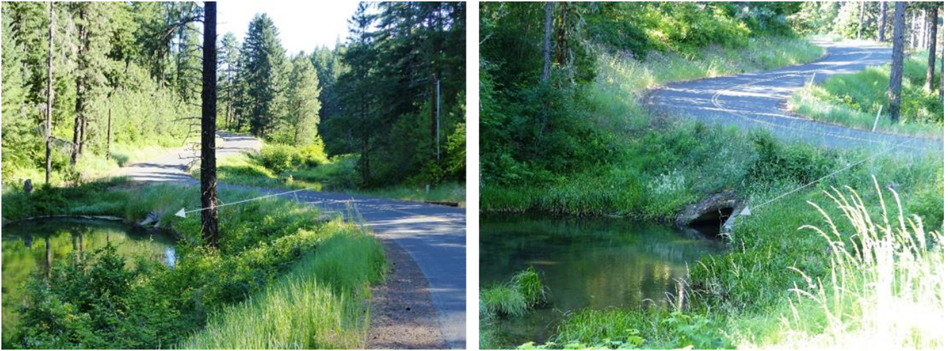
Figure 4: Spring Creek Road and Spring Creek culvert (L), close up of culvert outlet, upper end of pond and irrigation outtake (R).
