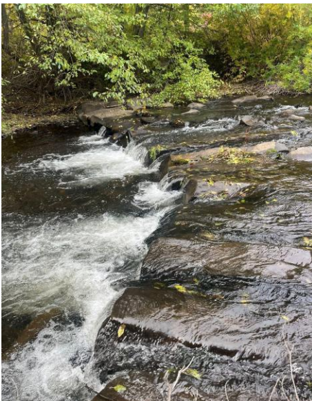
Figure 3. Photos of (A) Simplified channel confined against valley wall (from Reichmuth, 2007); (B) Example of one of the 15 boulder weir grade control structures built in 2000s
