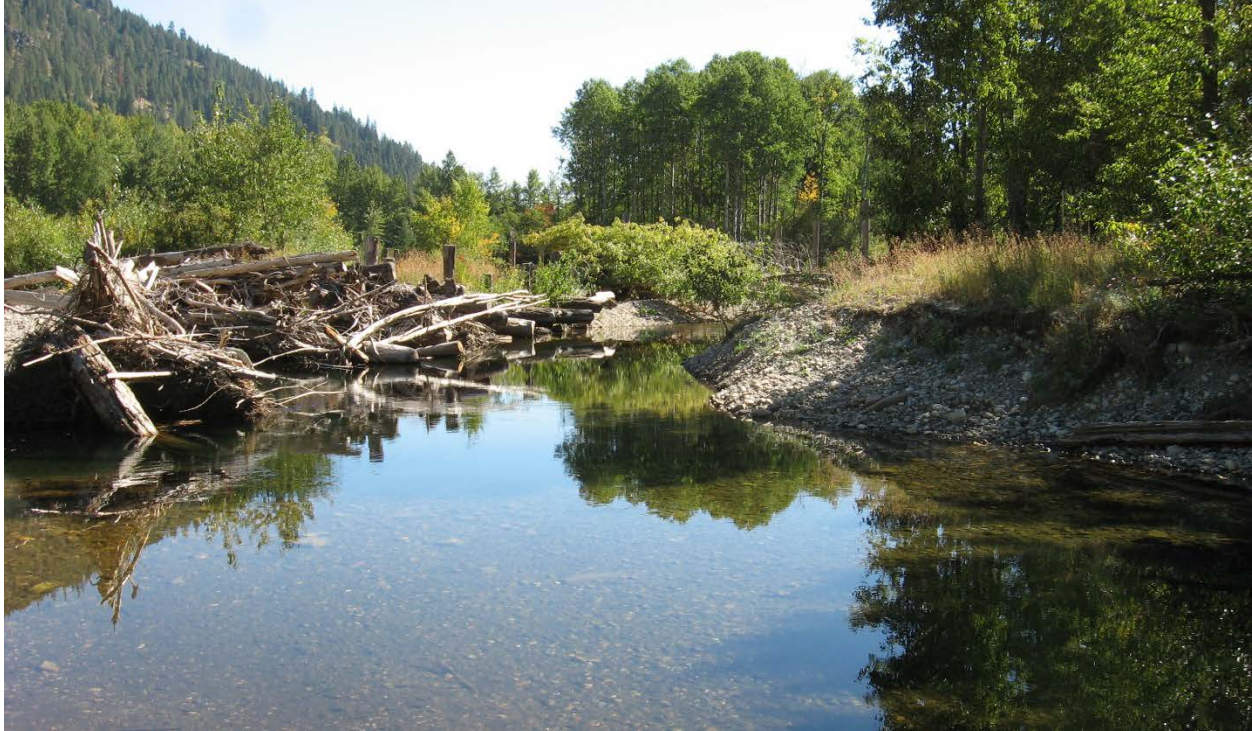
Figure 6. Example of inlet jam. Installed by Inter-Fluve 2013, photo taken in 2016 (Inter-Fluve).
