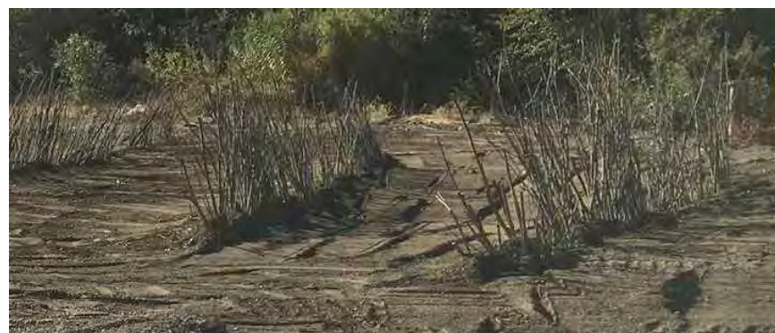
FINISHED WILLOW BAFFLES
