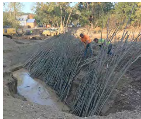
INSTALLATION IN PROGRESS
