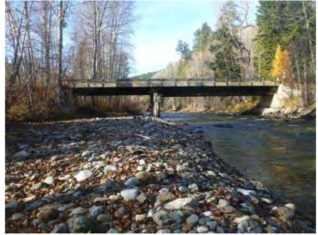
Figure 61. Bridge at RM 13.5 looking upstream.
