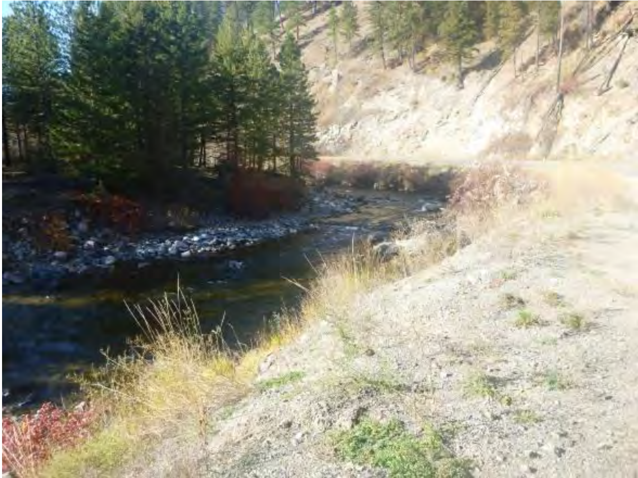
Figure 36 The road embankment at RM 9.15 looking upstream.
