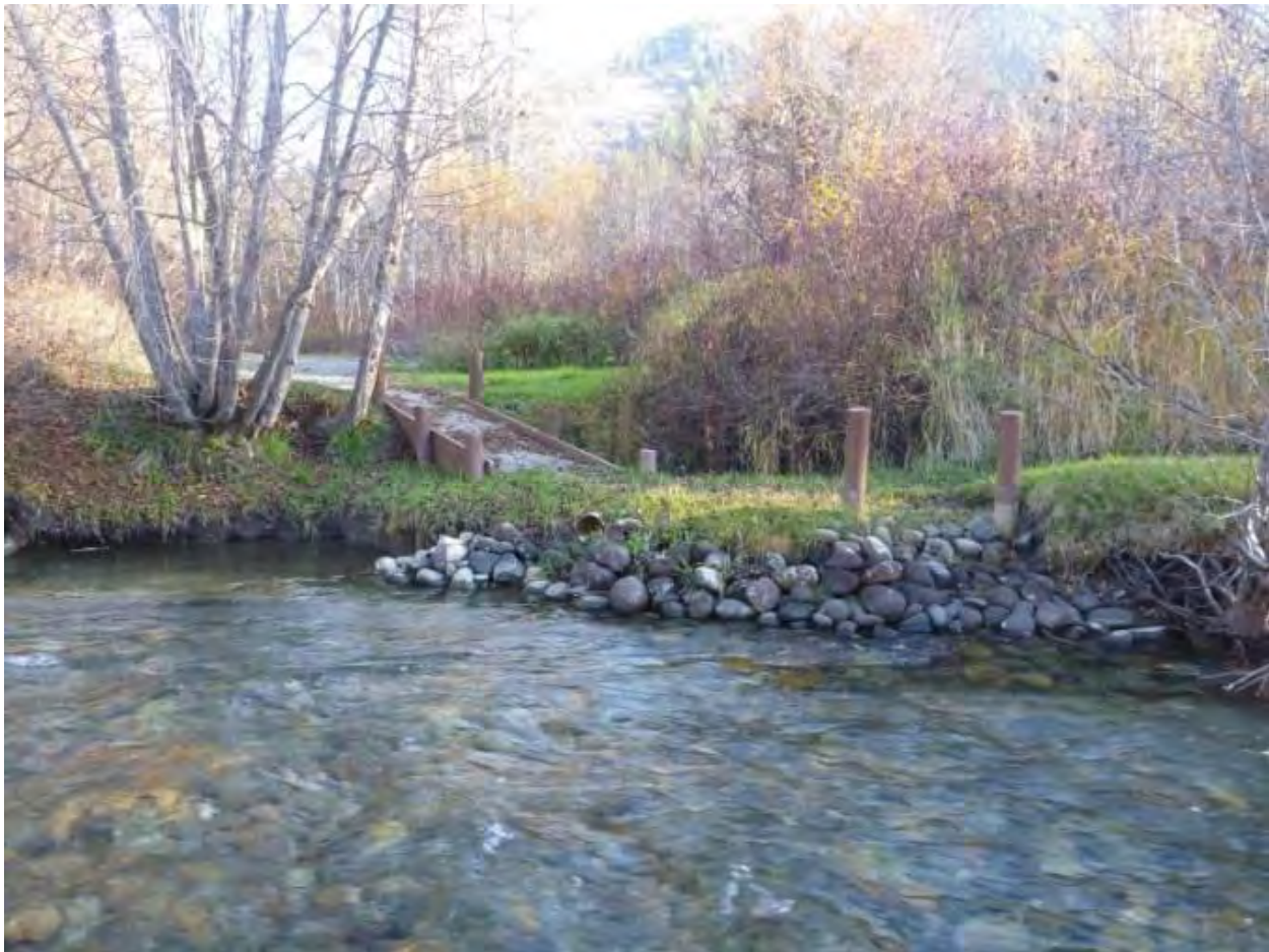
Figure 76. RM 13.8 riprap with large posts and a constructed footbridge constructed along river right opening to a gravel clearing.
