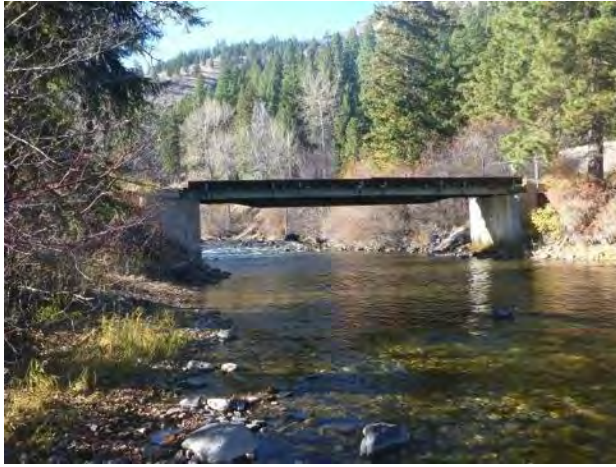
Figure 60. A small single lane bridge with abutments on the channel margin at RM 12.46.
