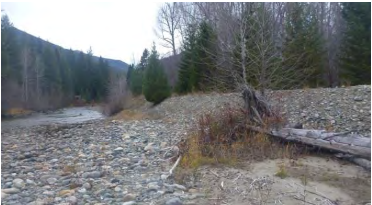
Figure 79. Pushup levee at RM 15.9 along river-left with established conifers
