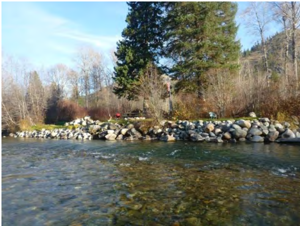
Figure 77. RM 13.85 Significant riprap has been placed along river right of this residential clearing with recreational elements up to the bank's edge.
