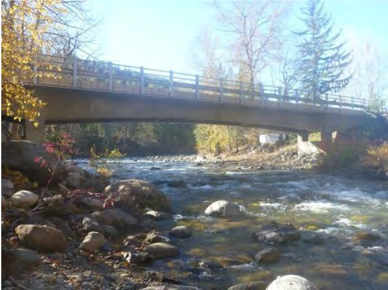
Figure 23 Looking upstream at the bridge at RM 8.4.
