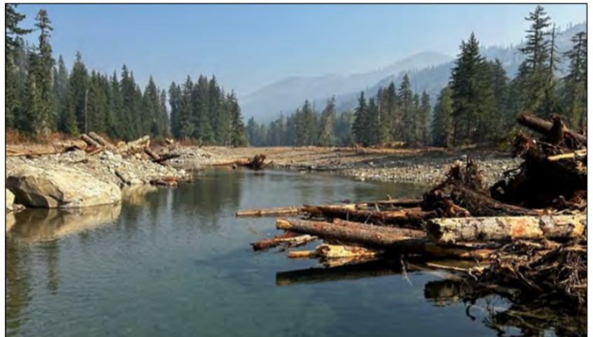
Side channel following creation, installation of habitat log complexes and engineered logjams, and planting. Photo taken following construction in fall 2025.
