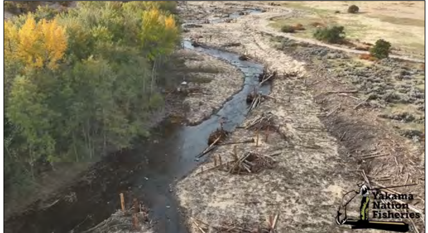
Above: Aerial view of log placements and reconstructed channels
