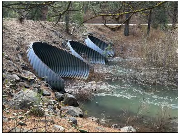
Brush Creek culverts before passage improvement
