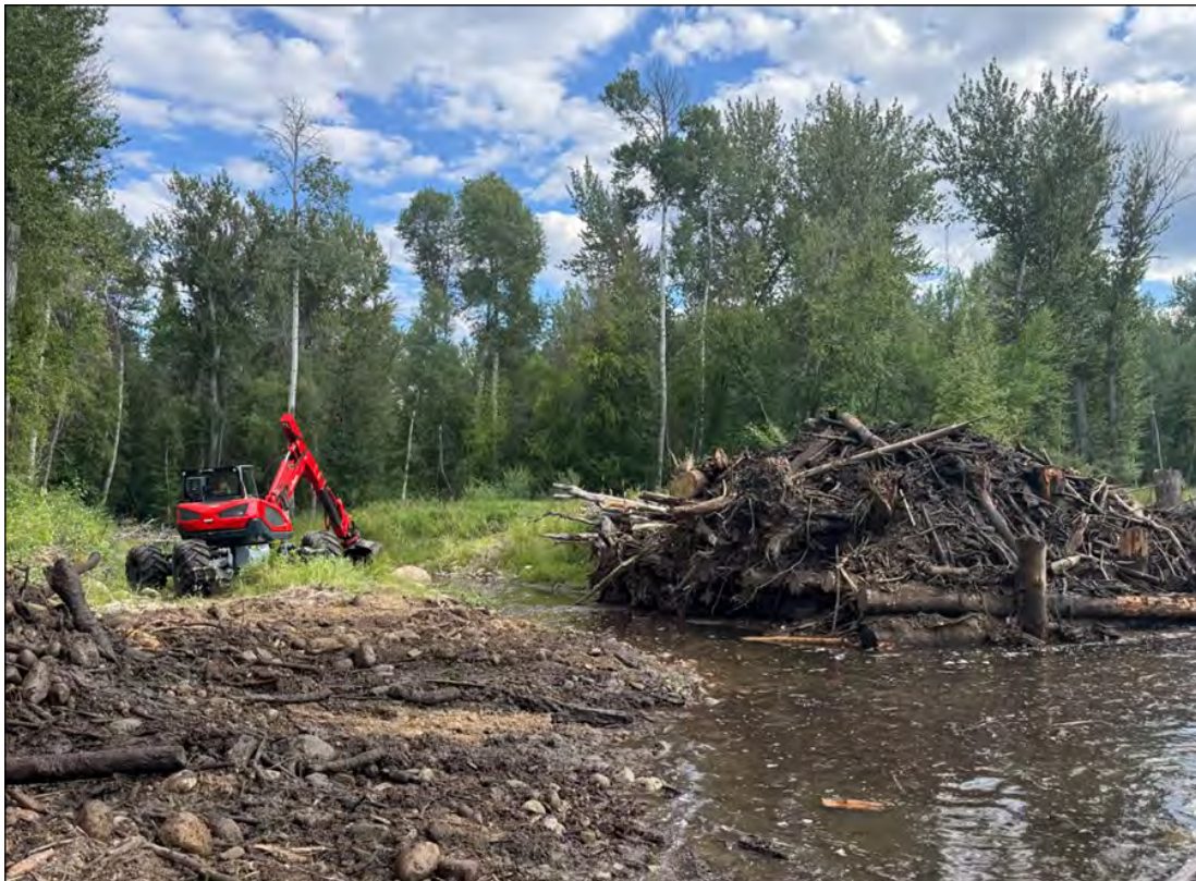
Low ground-pressure spider excavator cleaning out channel inlet.
