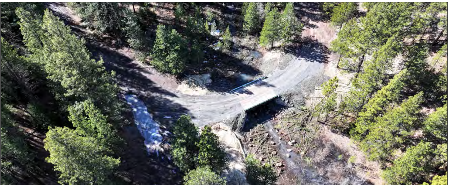
Aerial view, after full-span bridge replacement, restoring natural creek flow
