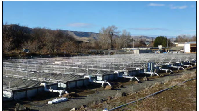
Above: Existing Raceways at Topxatuxt Hatchery
