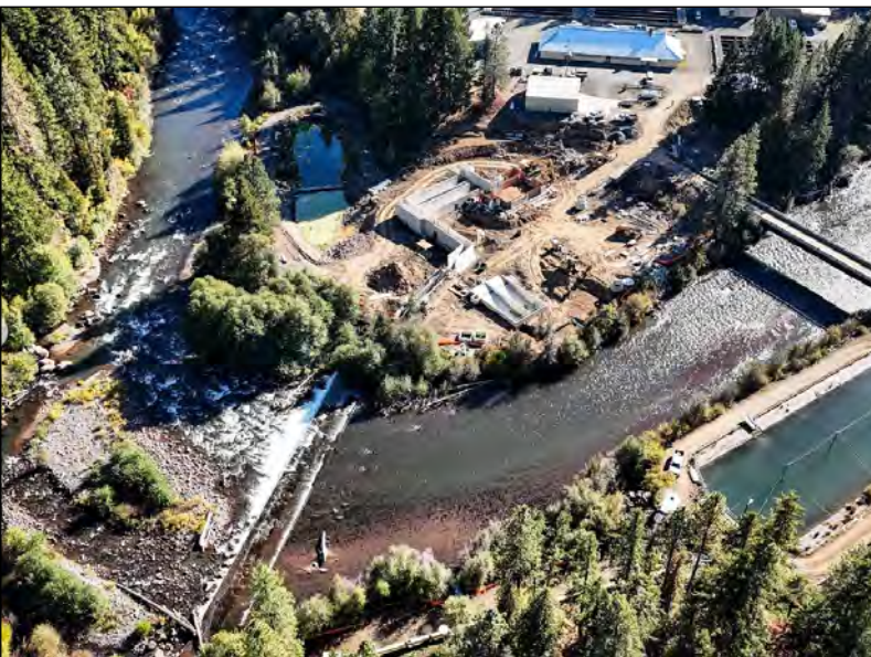
Above: Hatchery under construction, October 2025
