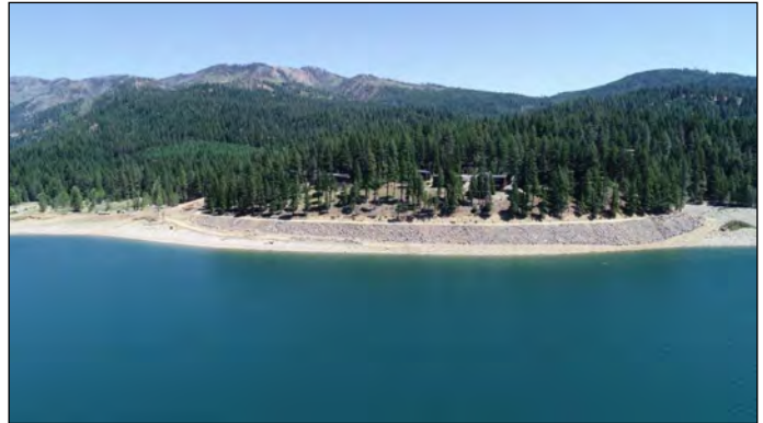
Timber Cove (during construction, summer 2025)
