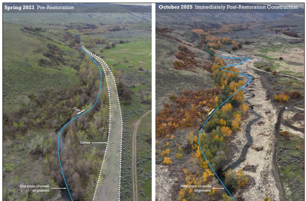
Above: 3-Way Levee Removal Project, Phase II, before and after construction
