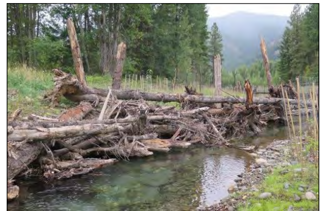
Fender Mill Alcove complex cover habitat in created pool
