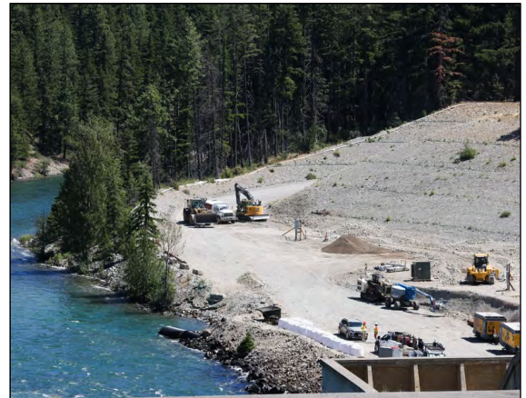
Above: Adult collector under construction below Cle Elum Dam
