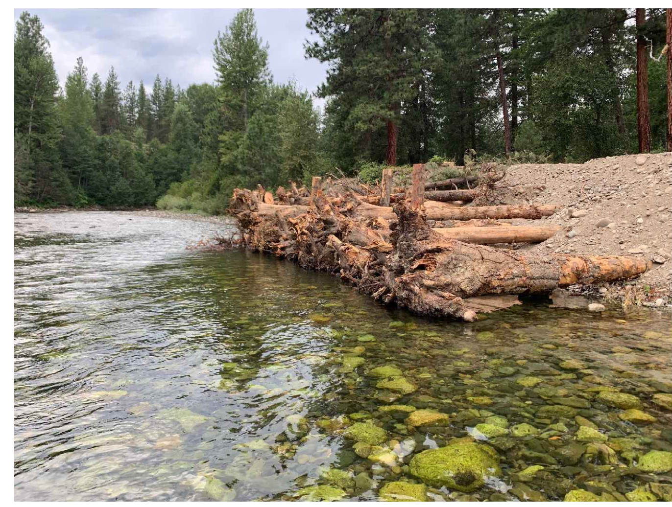
TYPICAL CONSTRUCTED BANK-BURIED LARGE WOOD STRUCTURE
