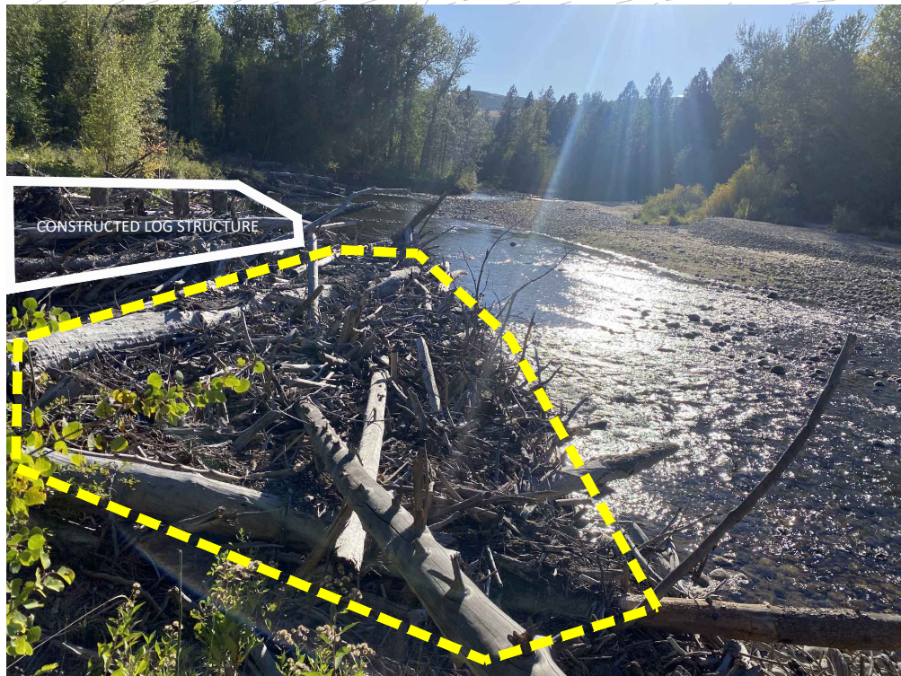
WOODY DEBRIS CLOGGING SIDE CHANNEL INLET
