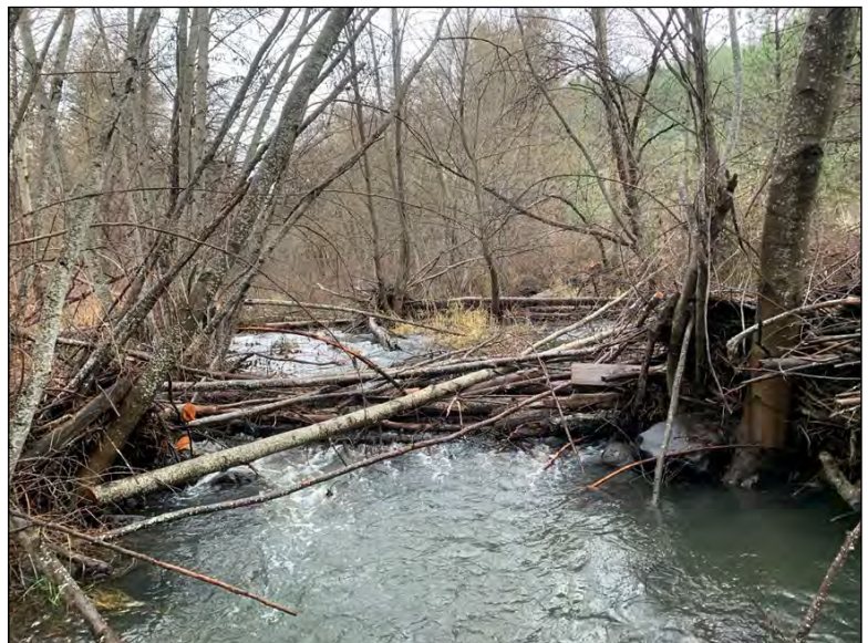
Above: Channel-spanning structure constructed at constriction point where wood has been naturally accumulating. Photo taken 12/12/23, under average Swale Creek winter flow conditions.
