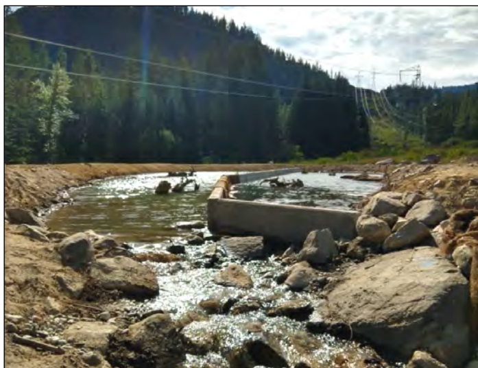
Above: Powerline acclimation site, Upper Nason Creek, final water test.
