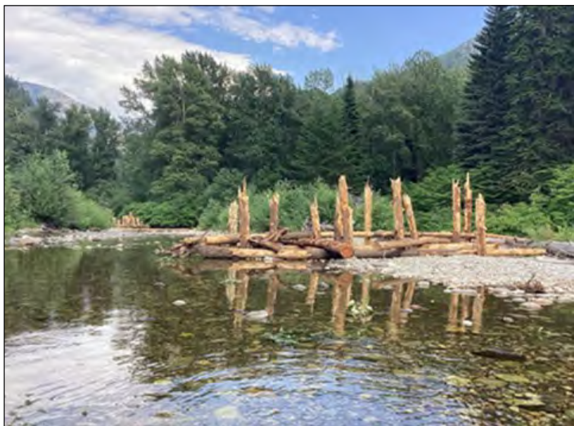
Above: Apex, cover habitat, and deflector structures. (YN)
