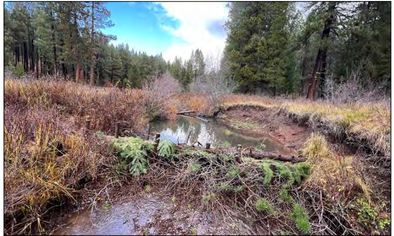
Above: BDA constructed in 2022 on Tepee Creek and maintained with addition of new green layer in 2023. Note – a side channel on the left, out of the photo frame, provides fish passage at a range of flows.
