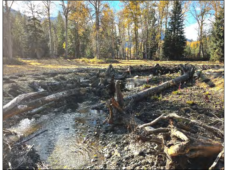
Above: Log structures installed to encourage pool formation and cover habitat.
