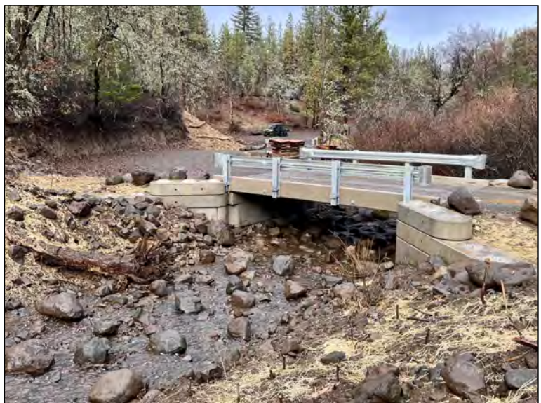
Above: New bridge installed to replace undersized culvert
