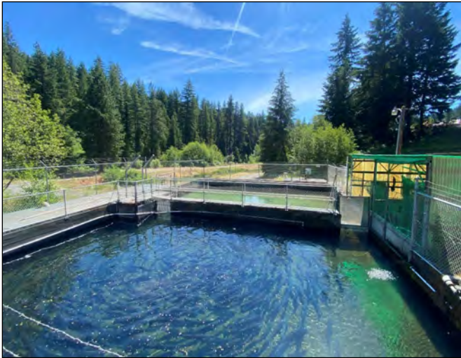
Above: Klickitat Hatchery facility.
