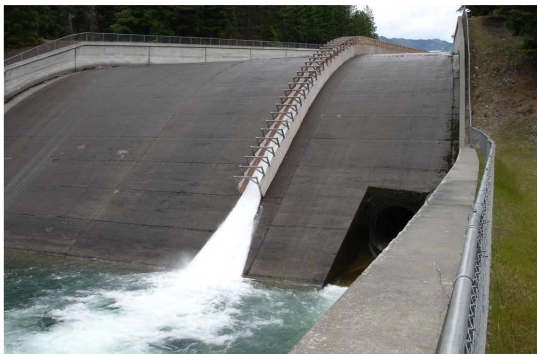
Cle Elum Dam juvenile passage structure
