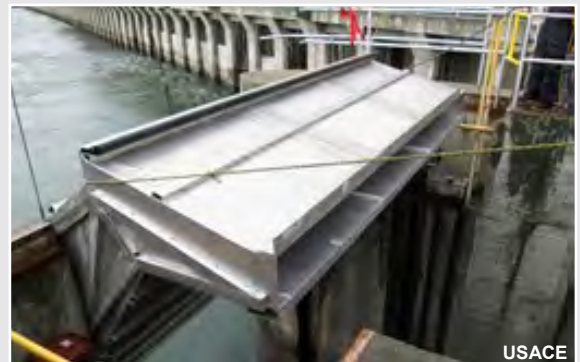
Lamprey ramp design and installation at McNary Dam
