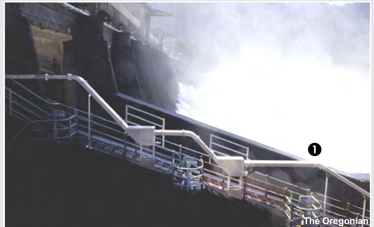
Lamprey ladder at Bonneville Dam
