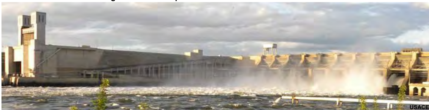
Juvenile bypass outfall at Ice Harbor Dam.
