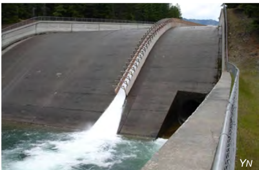
Cle Elum Dam juvenile passage structure
