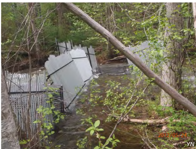
Kelt weir on Little Bridge Creek, Twisp Subbasin
