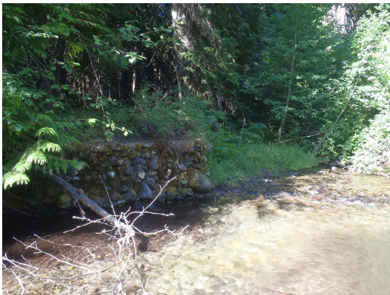
Figure 64. Remnants of an old bridge along SIDE25S.
