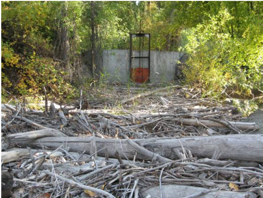
Figure 20. Headgate on river-left at RM 1.3 (October 2009).
