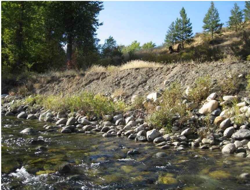
Figure 42. Erosion on river-left (north) bank near RM 3.2 (October 2009).
