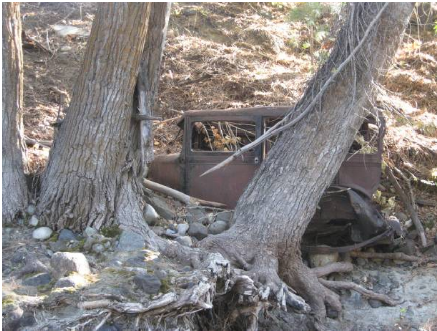
Figure 13. Old car bodies (“detroit riprap”) have been incorporated into streambanks in several locations (October 2009).
