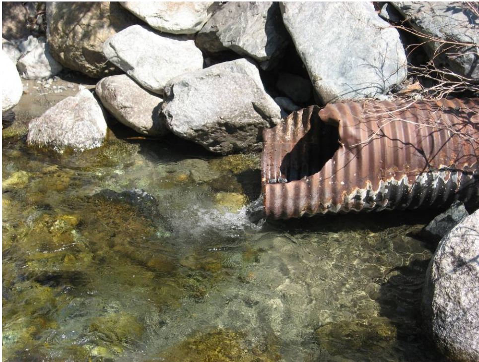
Figure 58. Culvert entering the mainstem on the river right bank near river mile 8.4.
