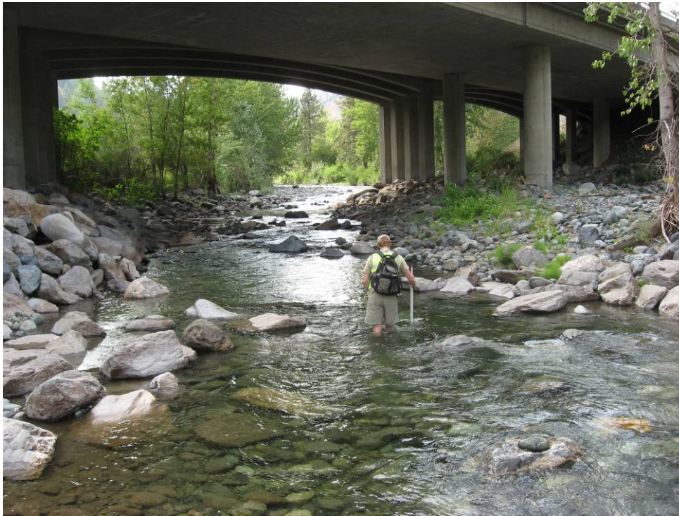
Figure 9. Hwy 97 Bridge at river mile 0.65.
