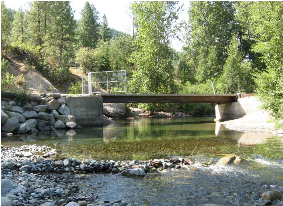
Figure 47. Private bridge crossing near river mile 6.5.
