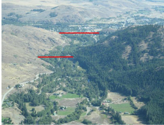
Figure 10. Low elevation oblique aerial photo looking downstream to the east at the transition between reaches T2b (foreground), T2a (mid-ground), and T1a (background) (September 2009).
