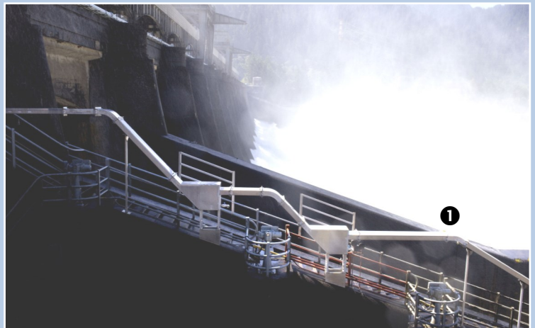
Lamprey ladder at Bonneville Dam
