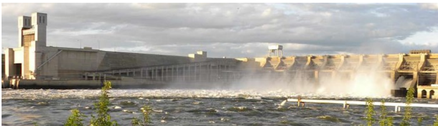
Juvenile bypass outfall at Ice Harbor Dam.
