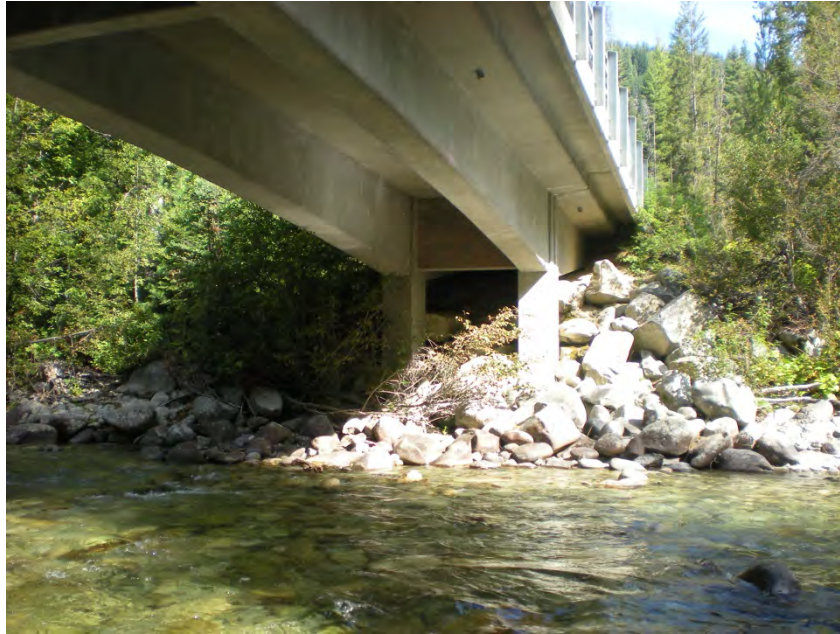
Figure 79. View of bridge abutment and bank hardening on river left near RM 31.85.
