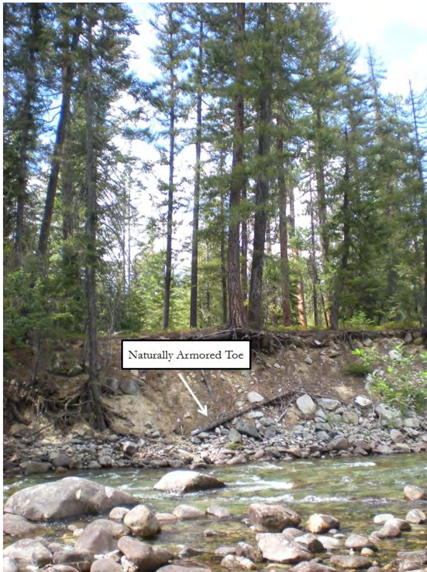
Figure 25. Naturally armored bank toe in confined portion of Upper Stillwaters Reach.
