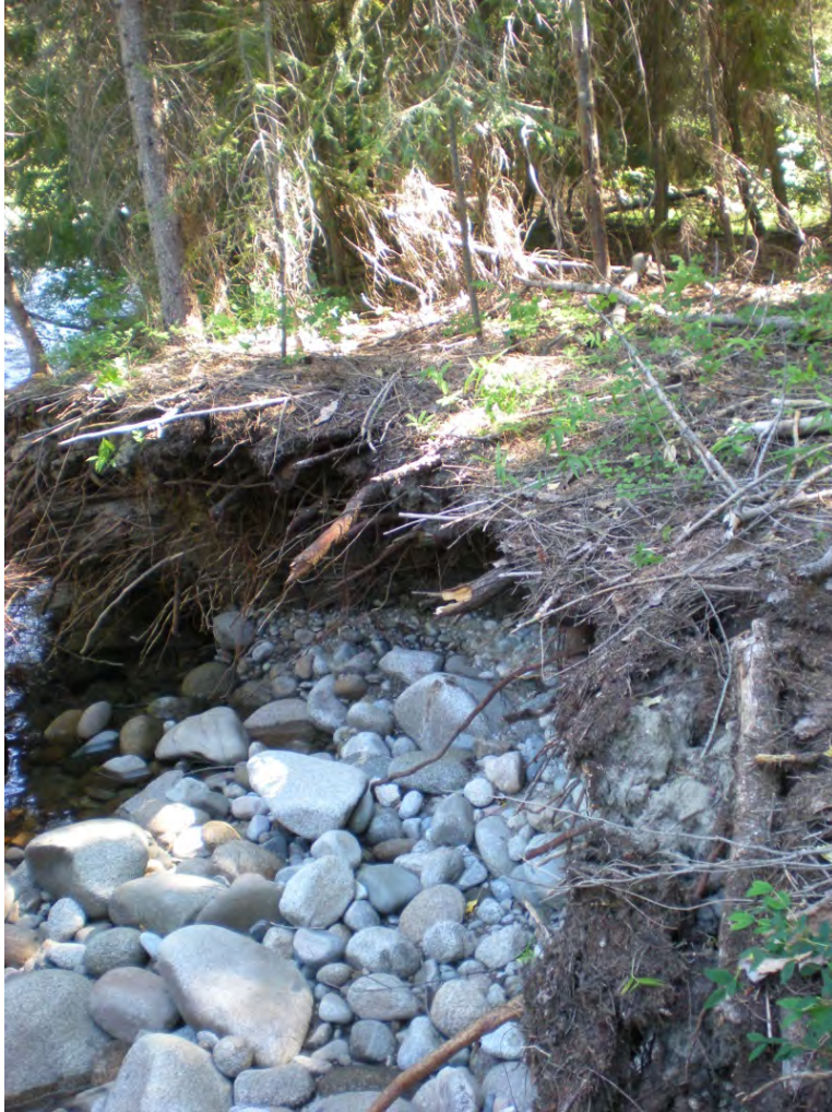
Figure 53. Undercut root wads along the right bank in Reach 10.
