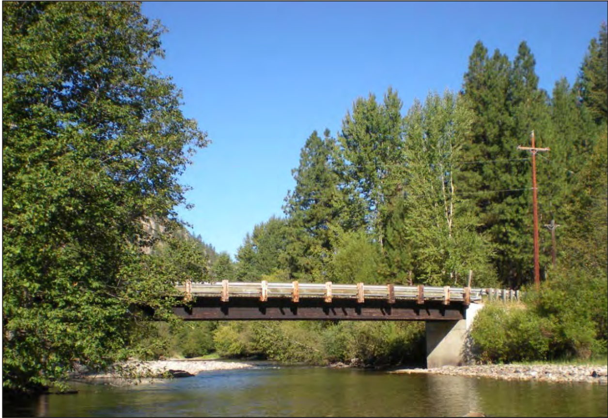
Figure 32. View looking upstream at the bridge crossing at RM 23.45. Bedload deposition (gravel bar) caused by backwater effects of the constriction, can be seen upstream of the bridge.
