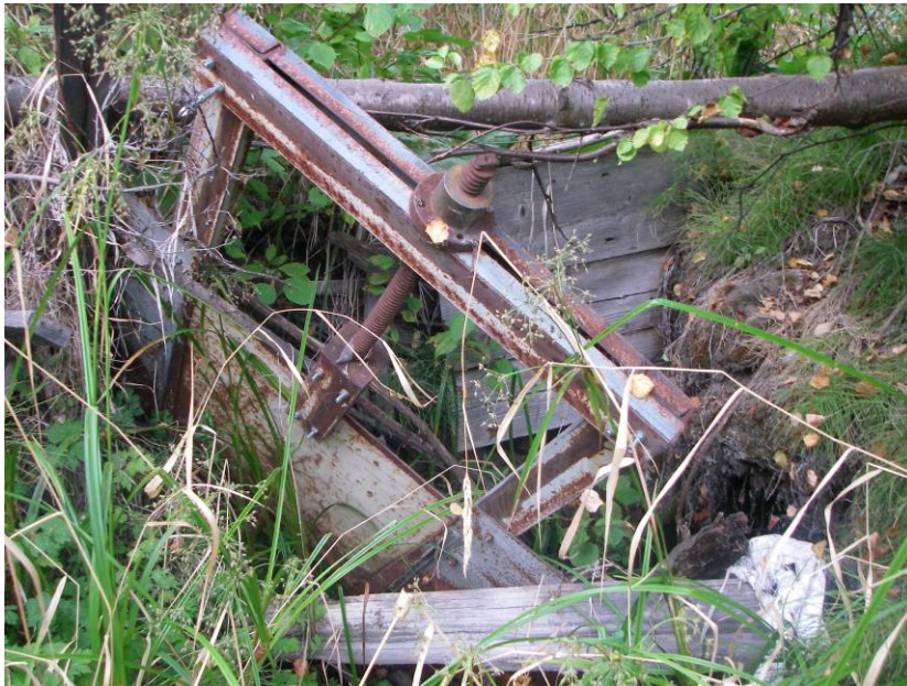
Figure 34. Headgate in an abandoned irrigation diversion at RM 0.7 (September 2011).
