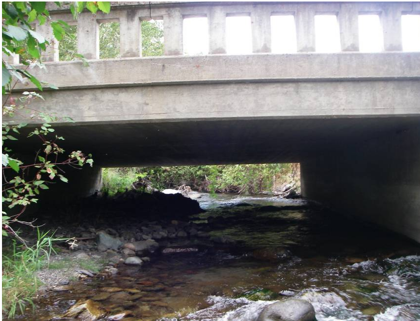
Figure 12. Habitat alteration and channel confinement at the Hwy 153 Bridge (RM 0.3).
