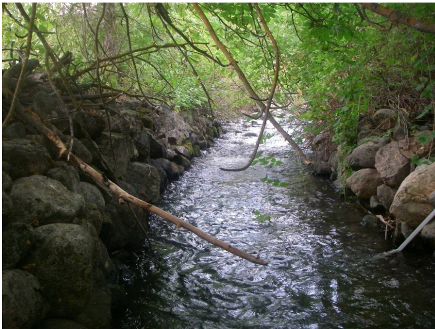
Figure 23. Riprap armoring limits floodplain connectivity and lateral channel dynamics near RM 0.3, Reach 1 (September 2011).
