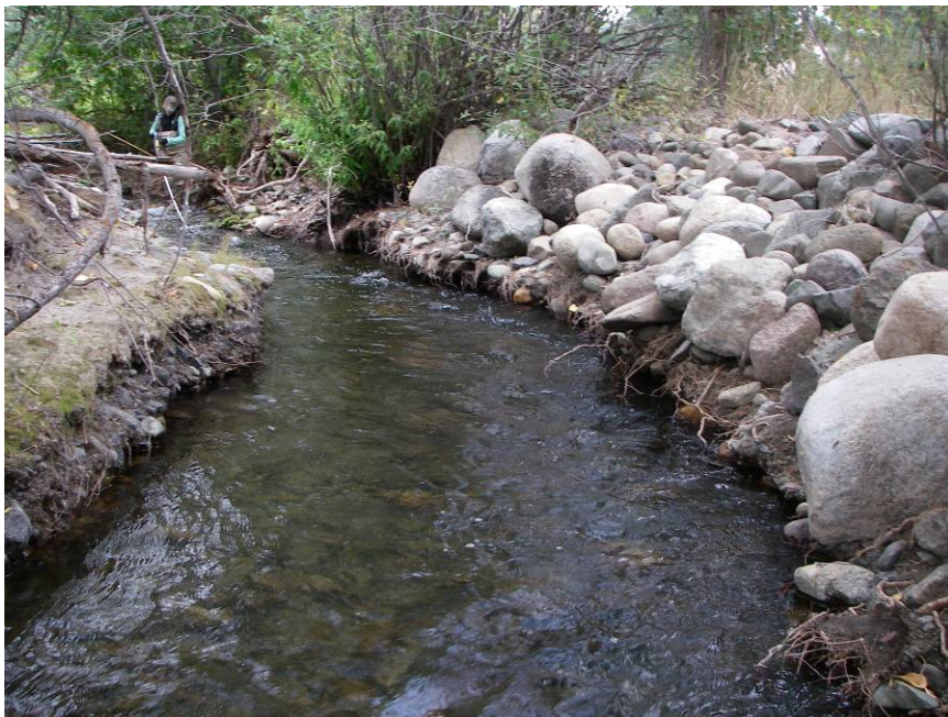
Figure 11. Bank armoring and scour along lower Libby Creek (September 2011).
