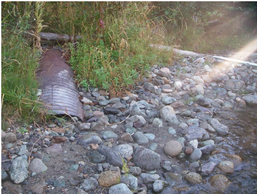
Figure 46. Remnant culvert in Reach 2 (September 2011). This culvert may have been used to drain the river-left wetland at RM 0.7.
