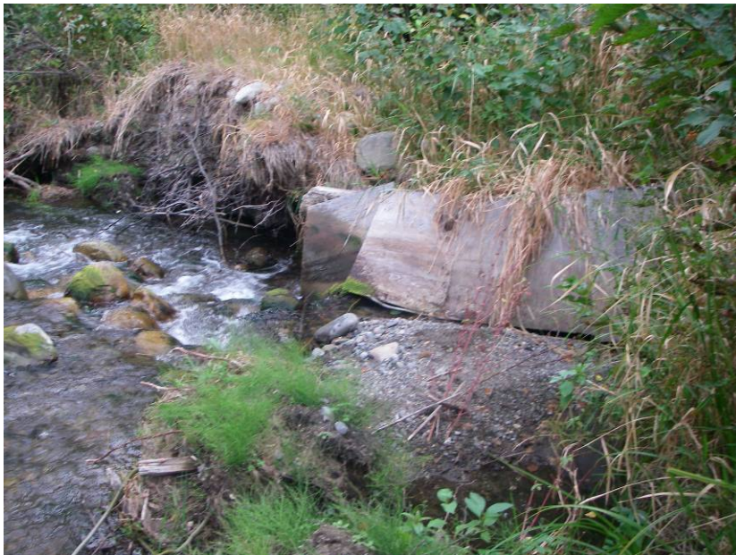
Figure 35. Plywood armoring along river-right near the downstream end of Reach 2 (September 2011).
