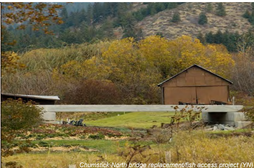
Chumstick North bridge replacement/fish access project (YN)
